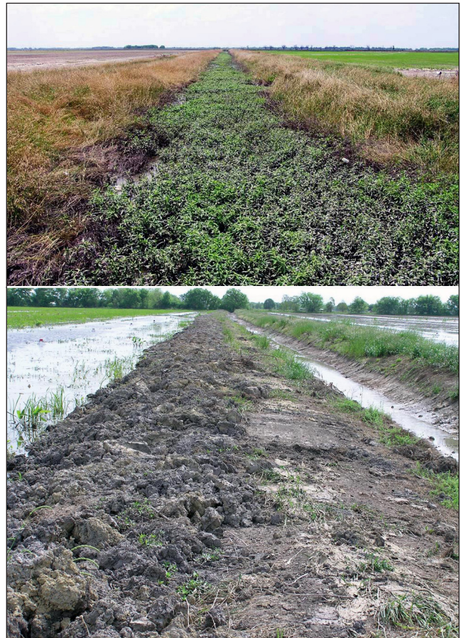
Sediments trapped in vegetated drainage ditches into which pond effluents are discharged can be used to rebuild or repair levees.
