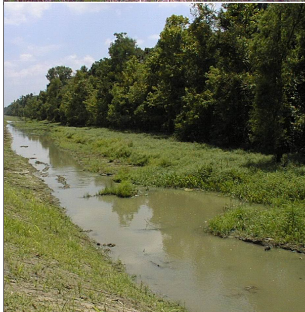
Suspended solids in effluent discharged from warmwater aquaculture ponds generally settled rapidly in drainage ditches, improving the quality of effluent before it entered receiving streams.
